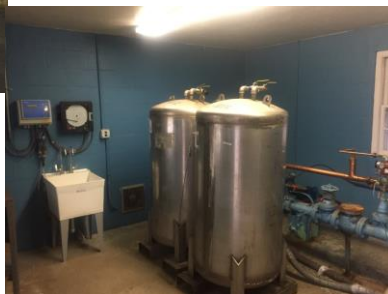
Anion exchange resin vessels at Well 10 →
