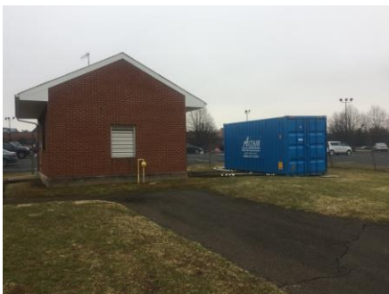
← GAC trailer at Well 17
