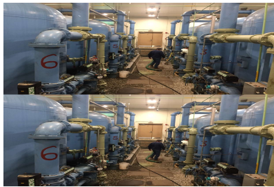
Grove Pond WTP
