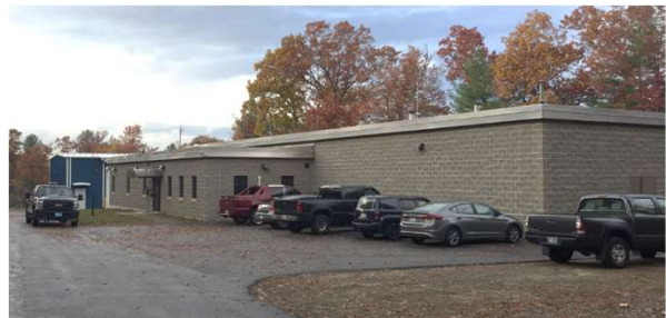
Grove Pond WTP
