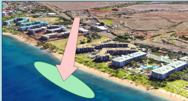
Kahului Wastewater Reclamation Facility
