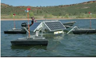
Utility 3 Solar Mixers
