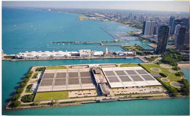
Jardine Water Purification Plant
